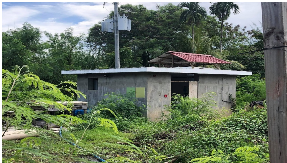
SPS 1, CIP Area (Unfinished under ICB-01, Rebid under ICB-05)
